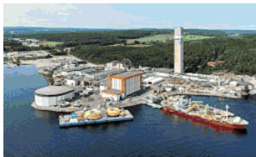
This factory in Halden, Norway, produces specialised cables for subsea interconnectors
