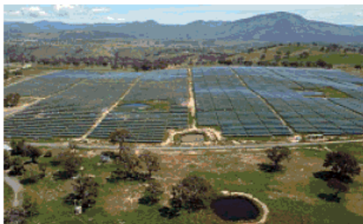
Williamsdale solar farm in Canberra, Australia
